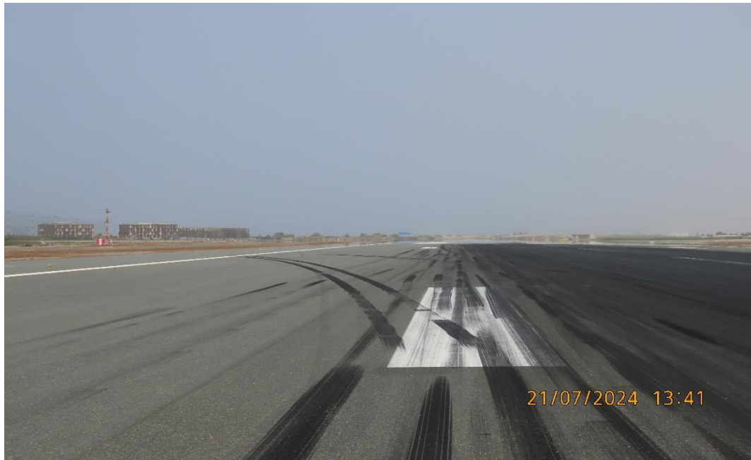
Figure 11: showing Left-Hand Main Undercarriage tire marks veering to the left of Runway 08L.
